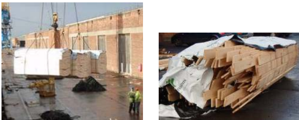
Figure 3.4.1 a) Sling lifting damaging packages b) collapsed, “barrelled” package
